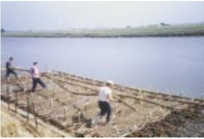
▲ A traditional fascine mattress construction along the banks of a tidal section of the River Great Ouse.
