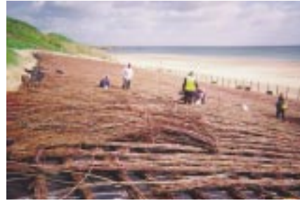
Fascine grid tied on to Geolon fabric prior to filling with brushwood.
