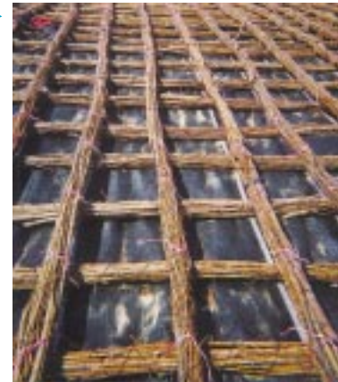
Fascine grid tied on to Geolon fabric prior to filling with brushwood.
