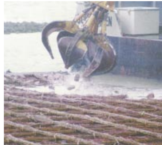
▲ Sinking a fascine mattress using rock placed with a crane
