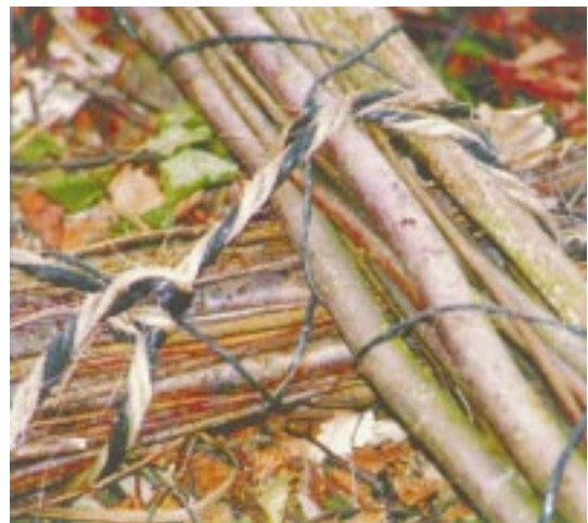
▲ Weips tied together to form the fascine mattress grid.
