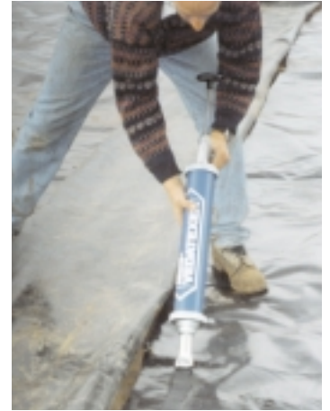
Sections that need to be joined can be done effectively using Vedatex sealant or double sided adhesive tape.
