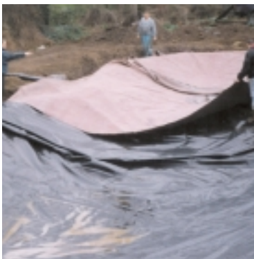
Installation of a MMG protection layer on top of a geomembrane.
