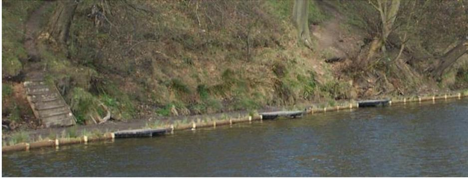
Vegetation can be encouraged by either sowing grass seed in the soil on top of the bank immediately behind the Nicospan and then covering with our Verdamat Erosion Control Matting or our Pre established Coir Fibre Pallets to increase protection and enhance the appearance of the slope.
