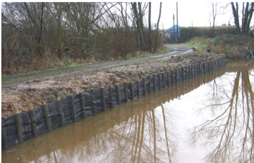
**Nicospan** is a product for vertical bank protection. It can provide a high-quality and very economical form of erosion control. Nicospan is a prefabricated, double weave revetment fabric made from strong UV stabilised monofilament yarns that are heat sealed to form a series of open pockets each having a width of 220mm so that 75mmØ/100mmØ posts can be placed into them.
