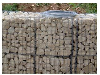
Gabions offer a time-honoured system for the construction of river walls - revetments – drainage channels - canals – reservoirs - coastal defences – retaining walls and many other applications.
