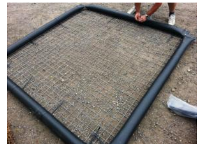
2. Place mesh base underneath booms and secure with heavy duty cable ties as shown
