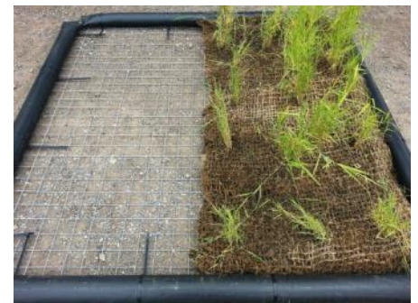
4. Place pre established coir pallet on to the island, preferably when the island is floating on the water
