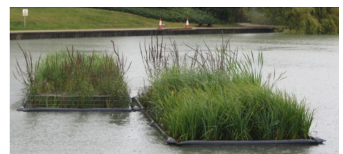
6. Your island is now ready to push in to place on to the water and then secure to the anchor weight
