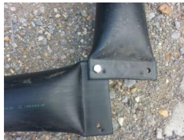
1. Bolt the corners together using stainless steel fixings
