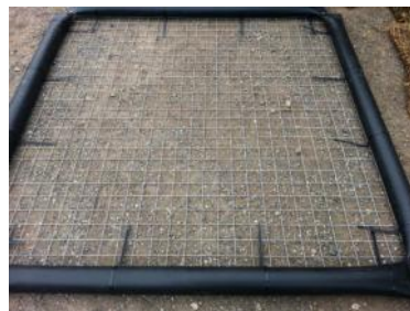
3. Your island should now look like this, bolted and tied in to place
